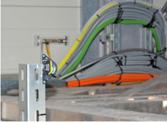
Photoelectric light sensors control the correct positioning of the pallets when entering the berthing space
