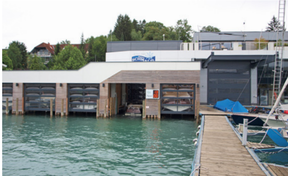
The new boat house in the Velden marina with the entrance to the BoatCube built on dry land
