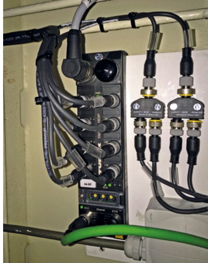
Control cabinets and other protective devices are no longer necessary with Turck's robust block I/O solutions with IP69K protection
