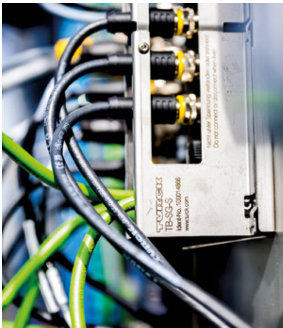
With the TB-SG stainless steel protective housings, almost all TBN I/O modules are also approved for use in ATEX zone 2
