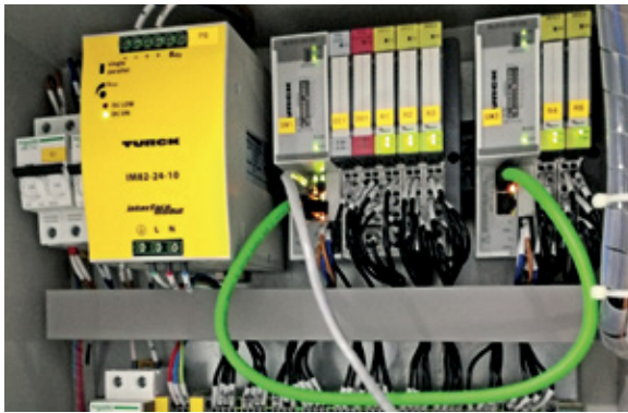
The BL20 RFID and I/O system from Turck ensures reliable communication with the PLC
