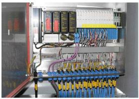
Ready to start: The fully installed excom station with redundant 230V power supply and fiber optic cable connector is ready to start up the plant.
