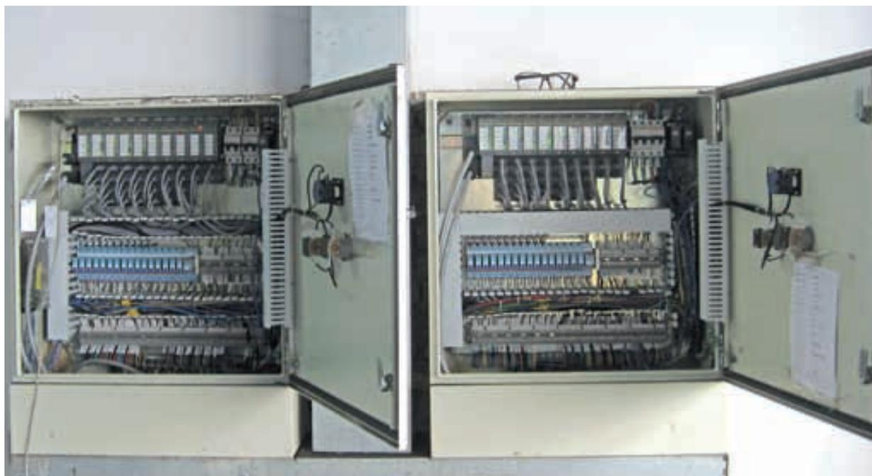
**A total of 14 BL67 fieldbus stations coordinate the DeviceNet data transmission between field devices and the higher level PLC by Allen Bradley**
