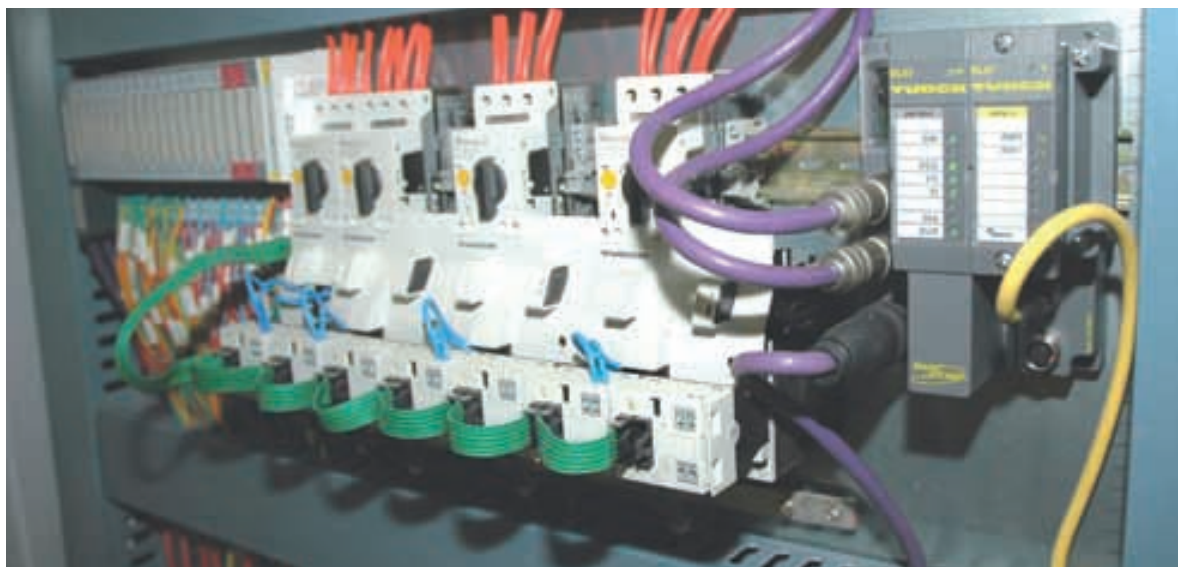
Turck total package: BL20 remote I/O system (l.), engine starter (m.) and BL ident Profibus Gateway (r.)
